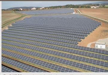
The BASE F/3 system is optimised for the range of framed modules. Installation in 3 rows onto the support construction is intended.
