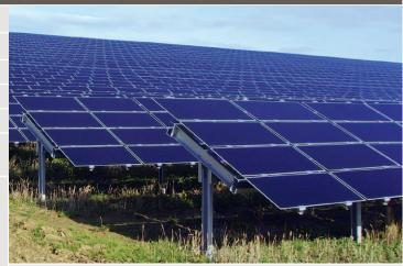
Perfect installation of the modules using separated GehrTec® laminate clamps, the lower part of which is fixed to a rail profile. In this way the frameless modules are positioned on the clamps which are fixed in the profile, and bolted. Thus we guarantee optimised installation processes for frameless solar modules.
